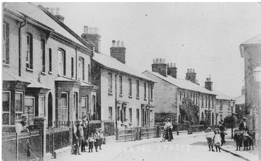
No 5 Chapel Street is on the extreme left
