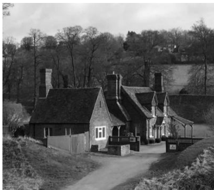
Caretaker's Cottage at Berkhamsted Castle – Soup Kitchen to the left
