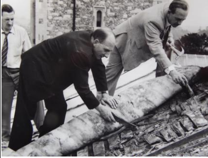
1958 – The Rector inspects the damage
